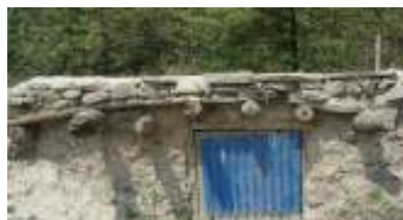
Figure 1. Underground apple storage
