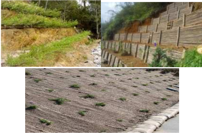
Figure 1. Bamboo Fencing (Source: Anil Gautam) 2. Jute Netting (Source: Sandbag) 3. Brush Layering (Source: LaRiMiT)
