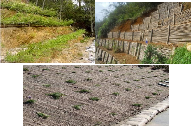
Figure 1. Bamboo Fencing (Source: Anil Gautam) 2. Jute Netting (Source: Sandbag) 3. Brush Layering (Source: LaRiMiT)
